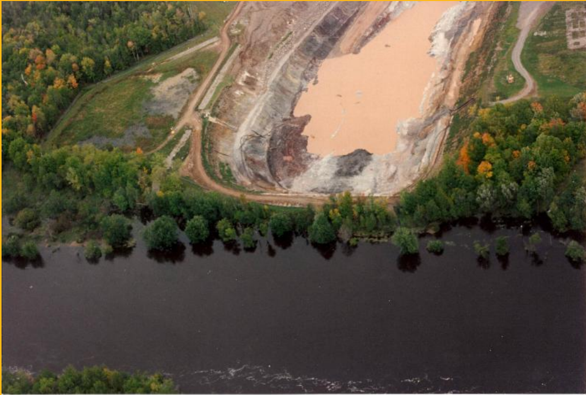
Flooding of the Flambeau River within 20 feet of the Flambeau Mine in 1994 Photo Credit: Bob Olsgard
